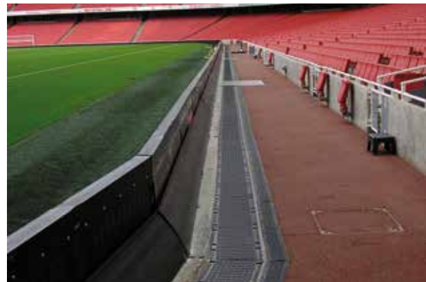
FC Emirate Stadium of Arsenal London with HAURATON SERVICE Channels
