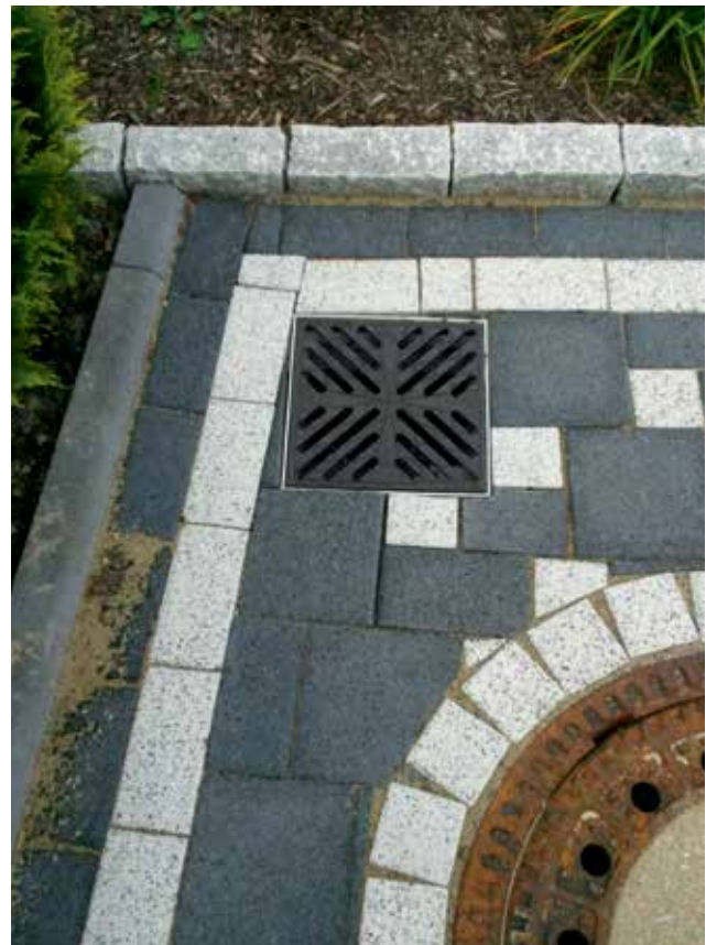
Private house in Wiehl, Germany
