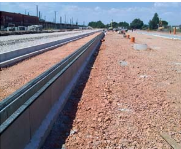
Easy installation due to integrated concrete runner
