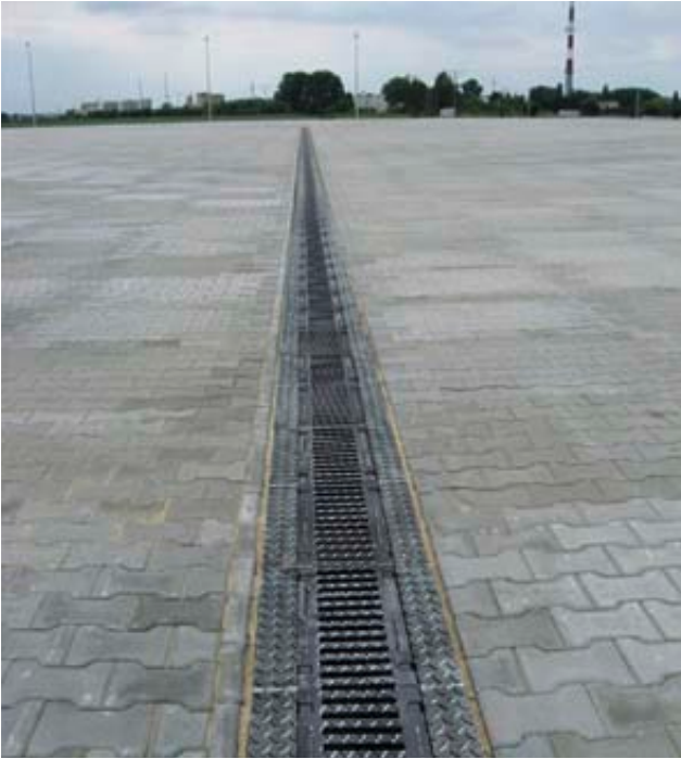
highest traffic safety due to 8-fold bolted grating
